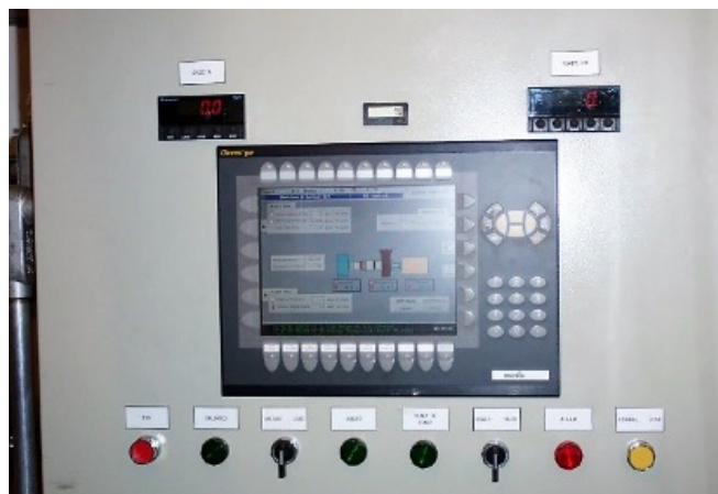
Control System Interface
